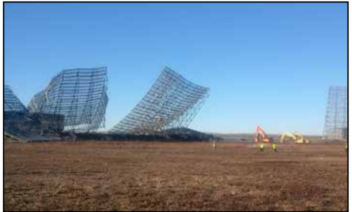
Removal of antenna arrays at Clear Air Force Station, Alaska.
